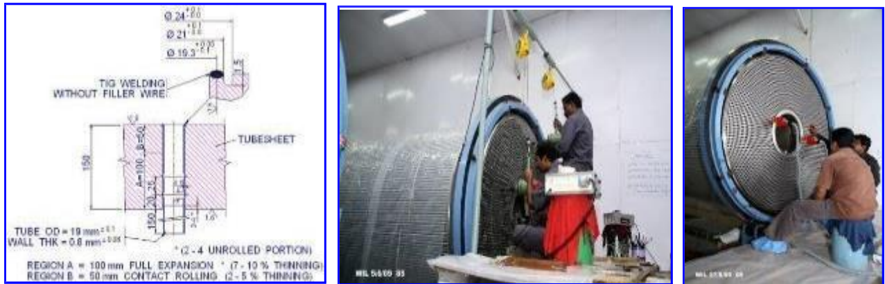
Figure 4: Tube to tubesheet rolling and welding of Intermediate Heat Exchanger
