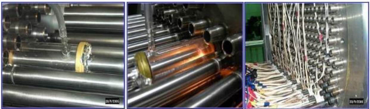
Figure.8: Tube to tubesheet welding of SG and local PWHT of joints
